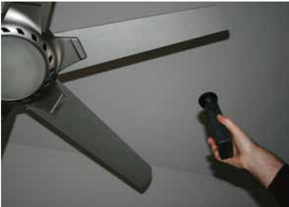
Checking Fan Speed and Balance
