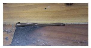
1. Cut the tip off of the caulk so that you can squeeze out a thin bead. Follow a few inches of the crack with a bead of caulk.
