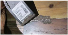
2. Use the putty knife to smooth the caulk over the crack.
