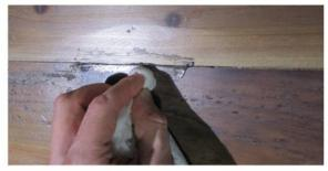
4. Use a damp rag to wipe the rest of the excess right up to the crack, then use a dry rag to wipe up the moisture from the wet rag.
